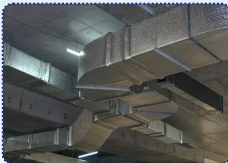
DUCT INSULATION
